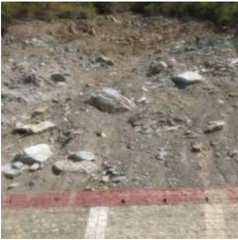
INITIAL STAGES DURING SITE HANDOVER BY CLIENT
