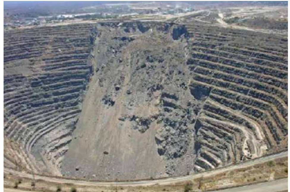
LANDSLIDE / INSTABLE SLOPES IN AN OPEN PIT MINE
