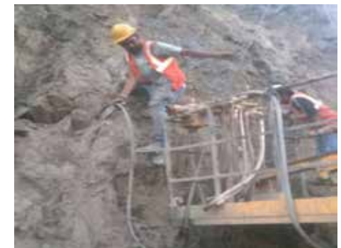
GROUTING BEING DONE
